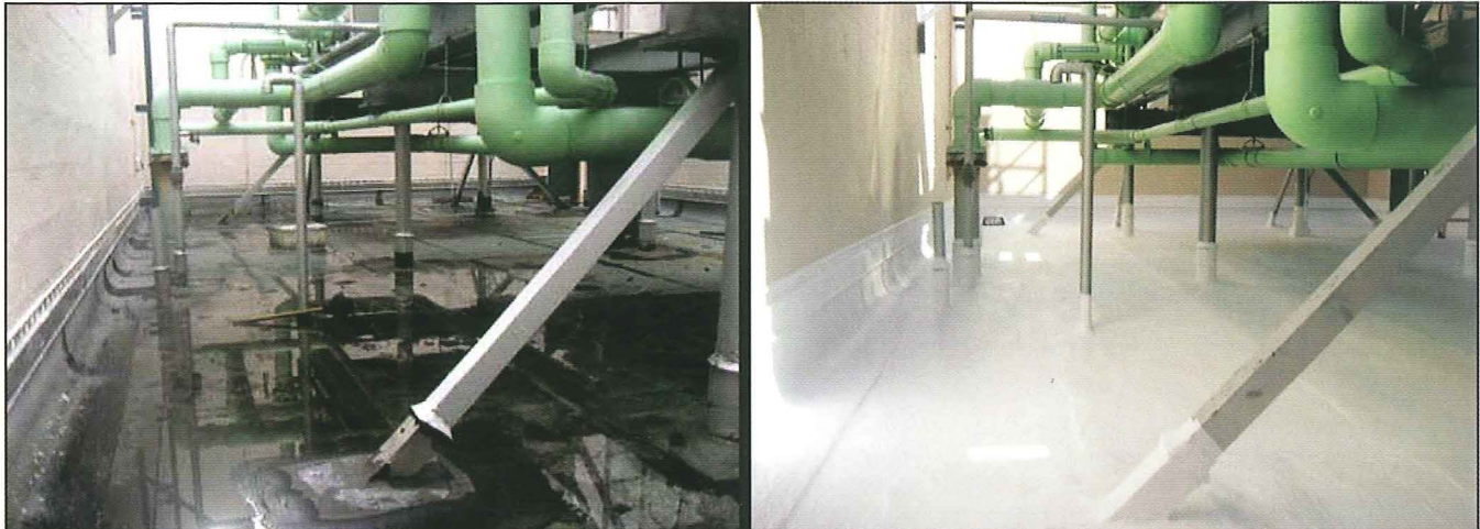
Leaky, failing asphalt substrates are converted to seamless, sustainable cool roofs.
