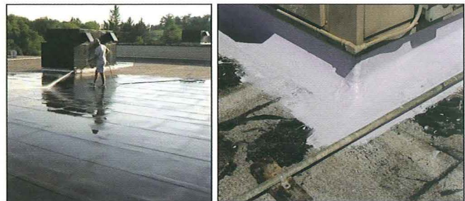
Power wash; seal curbs and penetrations
