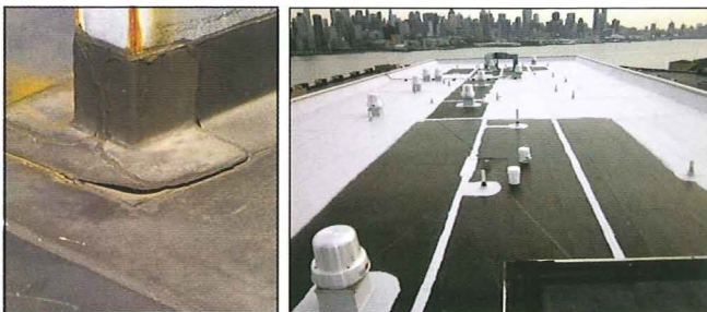
Seal all seams, splits and penetrations
