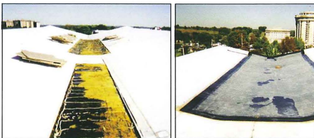
Repair substrate integrity as necessary
