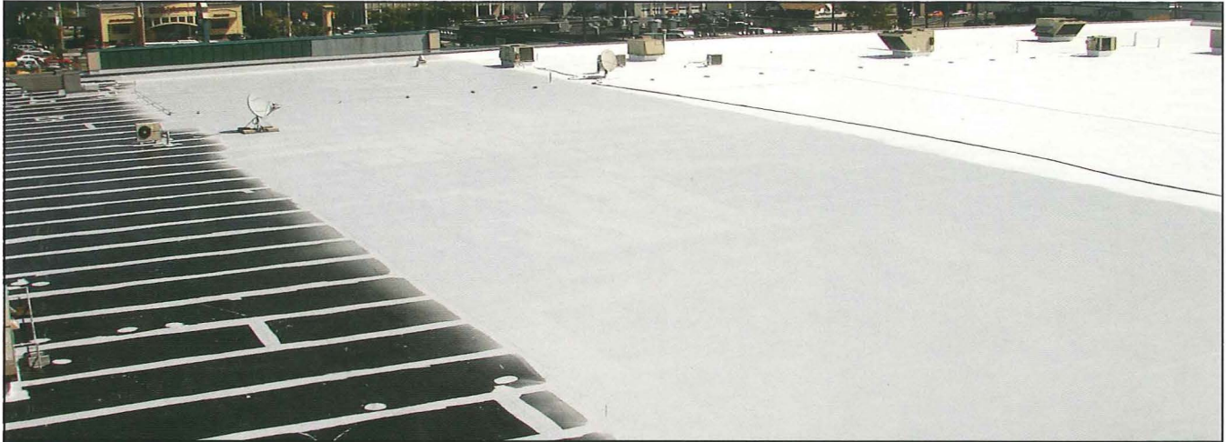
This failing single ply substrate is converted to a seamless, sustainable cool roof
