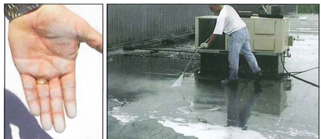
Clean surface and neutralize chalking
